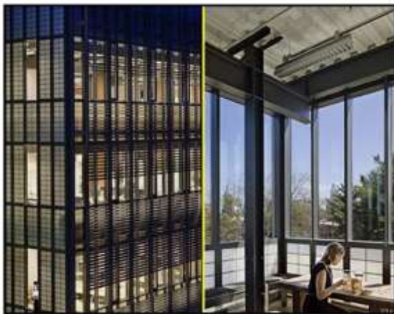
Fig. 19. A facade application of aerogel at the Yale University Scripps Building and Gallery [108].
